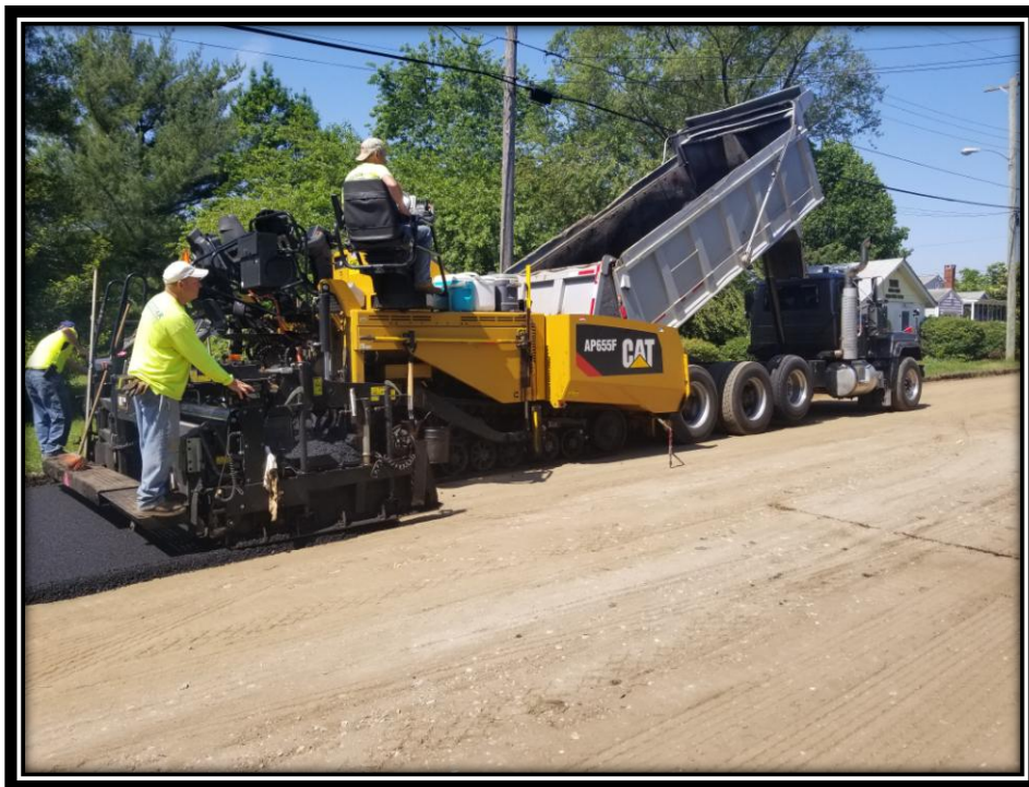
Figure: 3 – Installation of HMA 19M64 base course on Joffre Avenue
