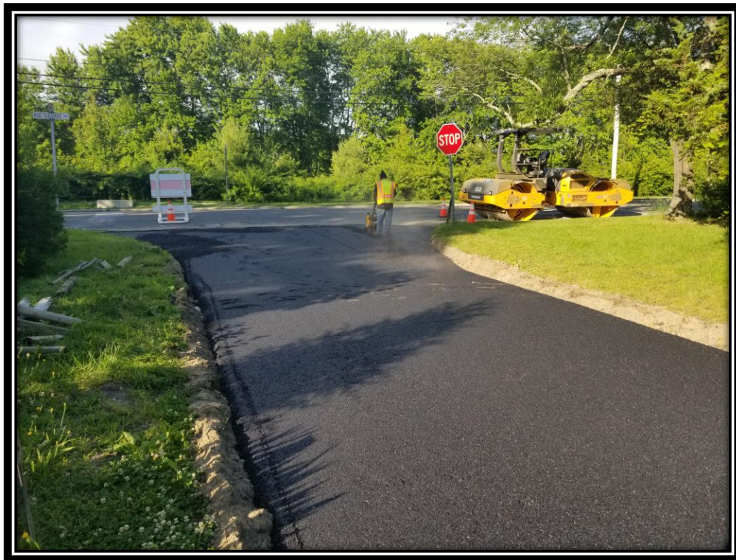
Figure: 1 – Installation of HMA 19M64 base course on South 2 nd Street
