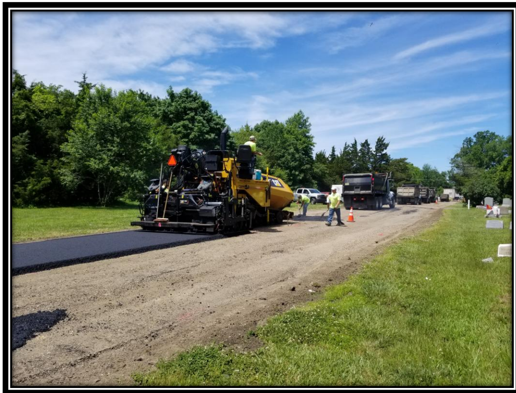
Figure: 3 – Installation of HMA 19M64 base course on Church Street
