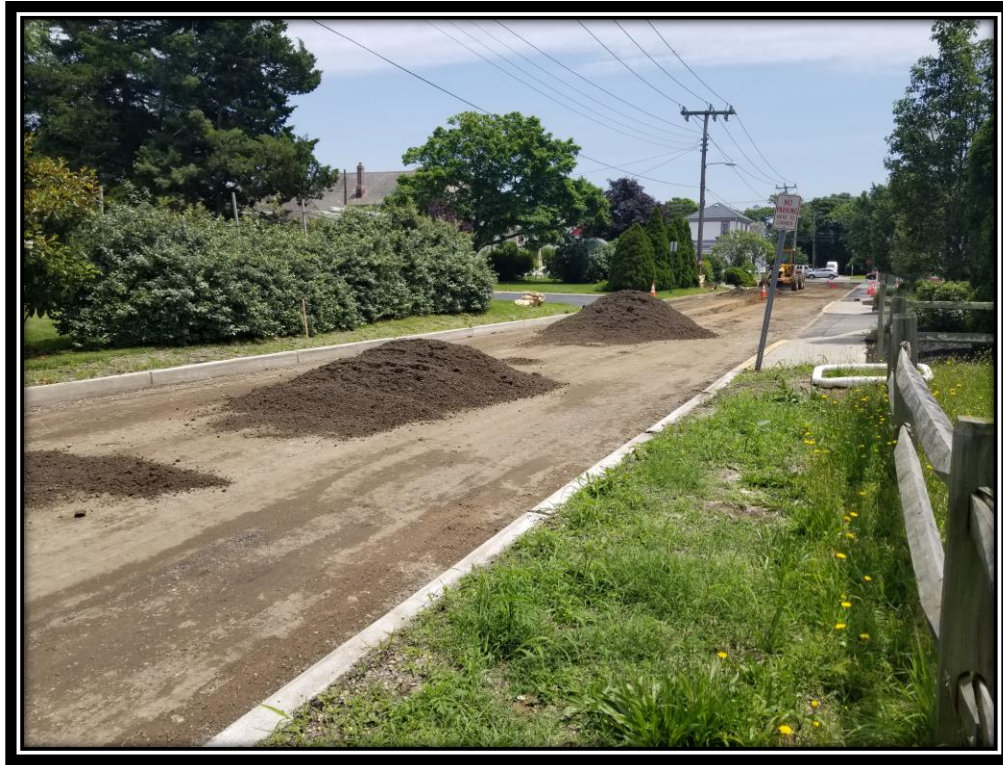
Figure: 2 – Installation of dense graded aggregate on Church Street
