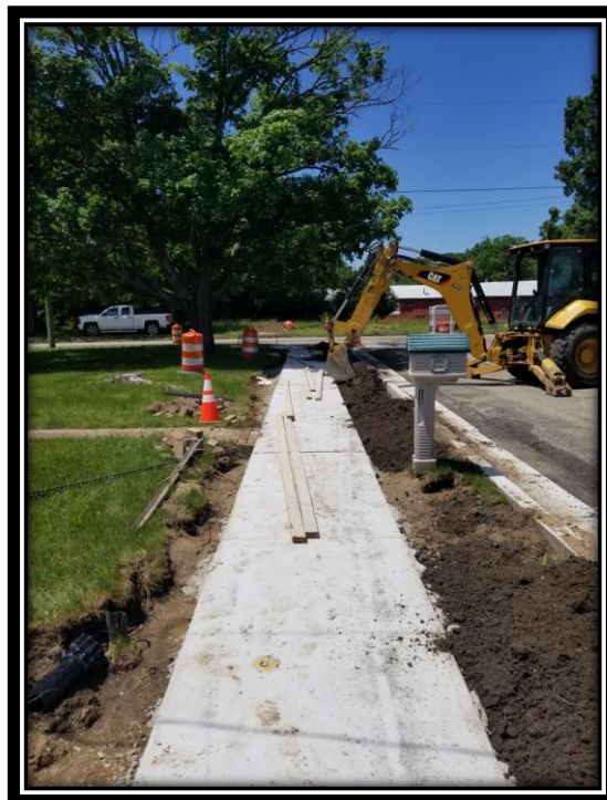
Figure: 3 – Topsoil restoration along the newly installed concrete sidewalk and curb & gutter on West Atlantic Avenue along the eastbound lane between Front Street and South Boyd Street
